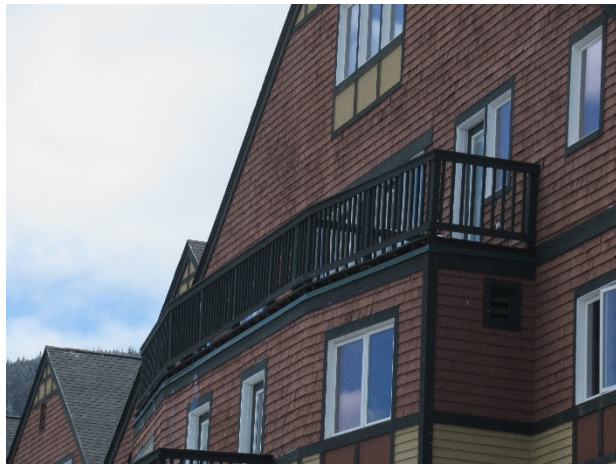
Balcony at flat roof
