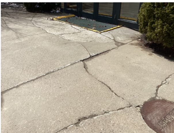
Sidewalk cracks
