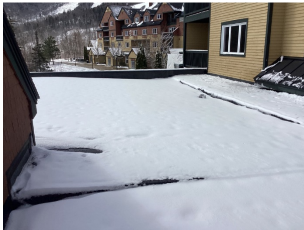
Flat roof overview
