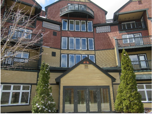
Wood siding overview
