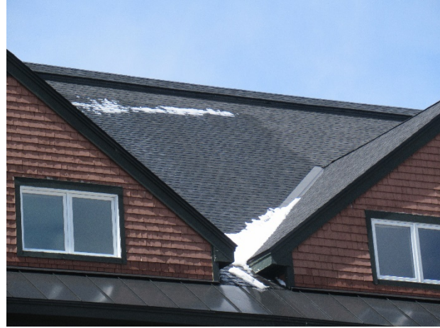
Replaced roof overview
