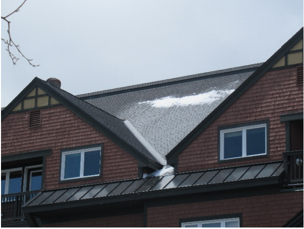
Replaced roof overview
