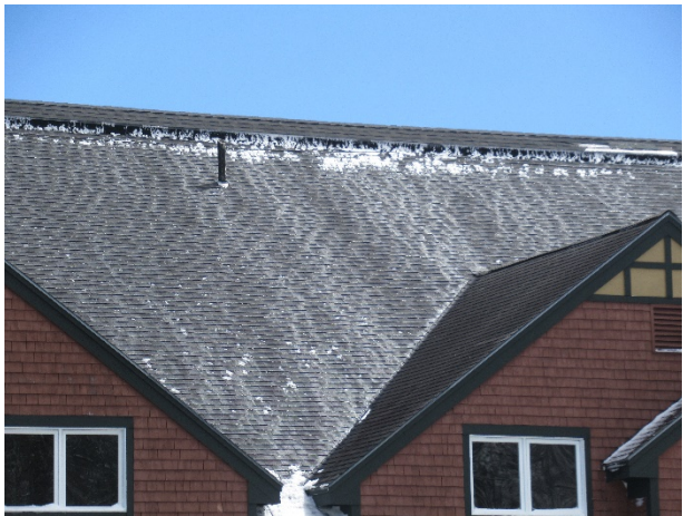
Replaced roof overview
