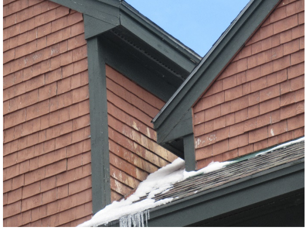
Finish deterioration
