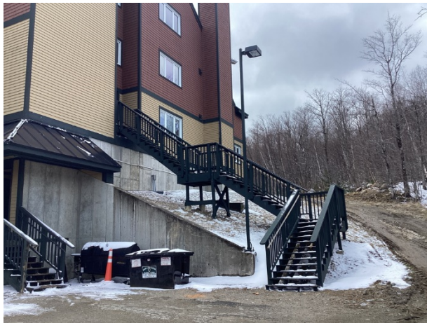
Light pole and fixture
