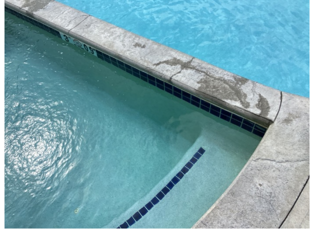
Pool plaster finish with tile perimeter
