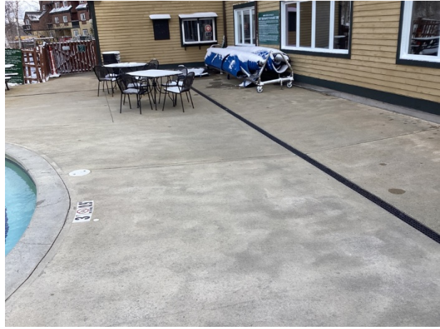
Concrete pool deck overview
