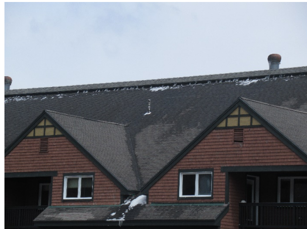
Remaining original roof section
