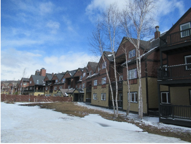
Rear elevation overview
