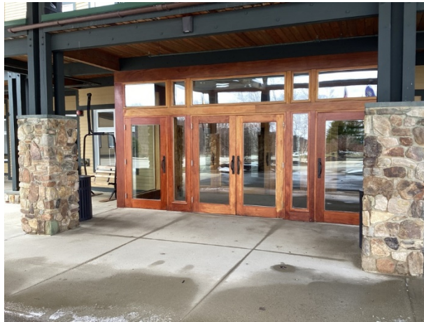
Main entrance doors
