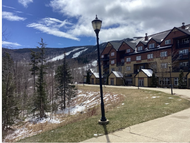
Leaning light pole and fixture
