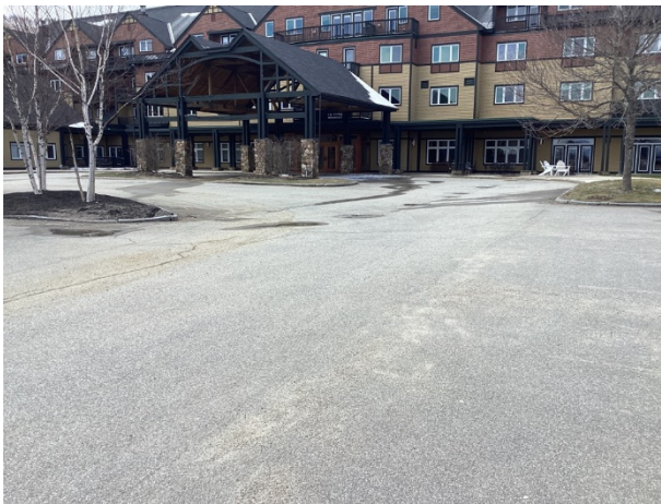
Entrance driveway and parking area overview
