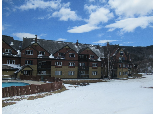
Rear elevation overview
